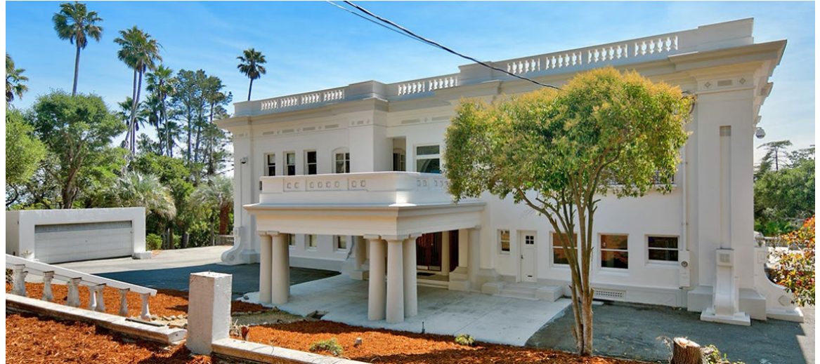
Spring Mansion and existing garage
